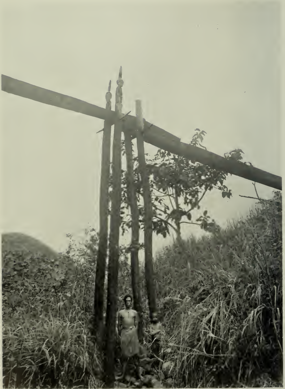
Aqueduct across the Davudavu creek (Bartle Bay) showing carved figures on posts
